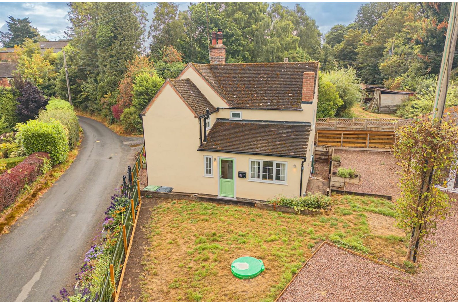
Pool House Hill Pool, Chaddesley Corbett DY10 4NL
